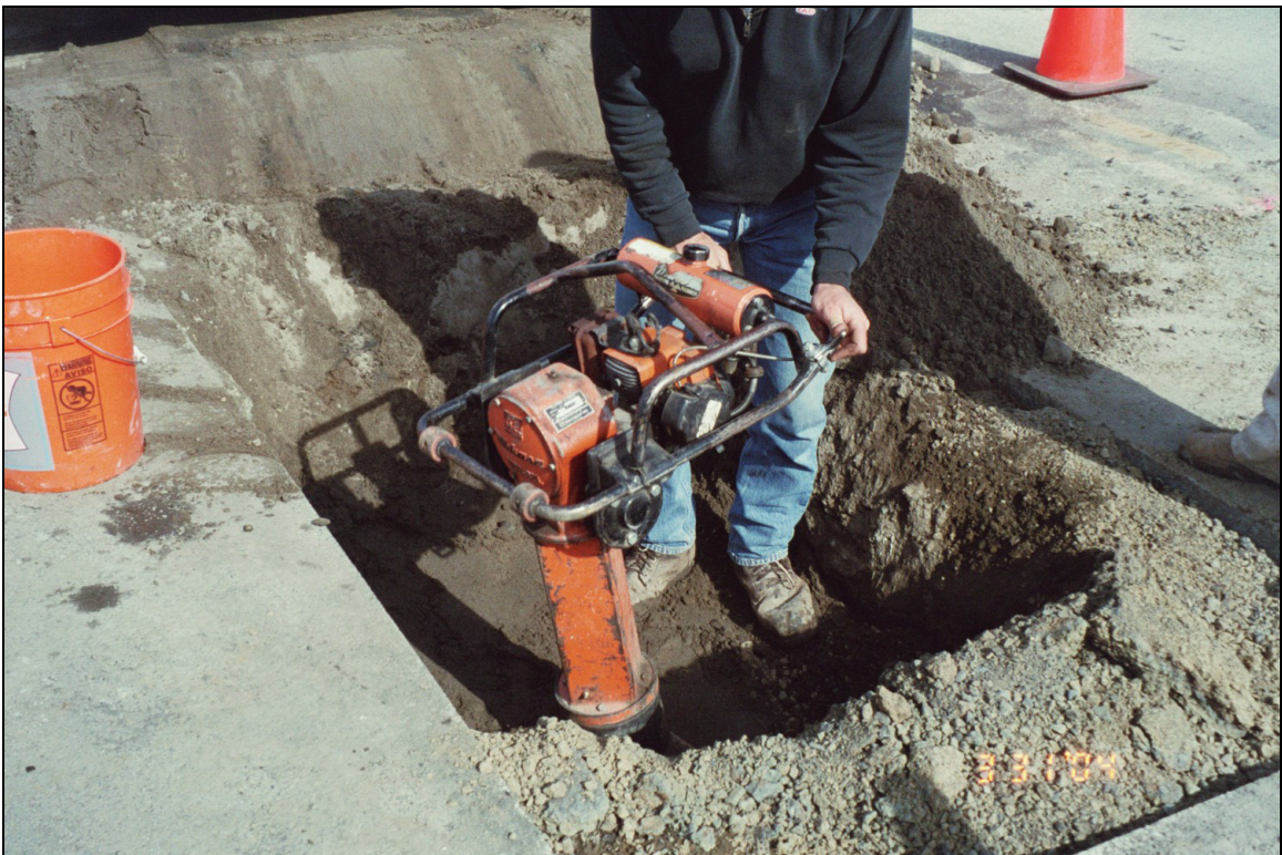
Photograph 14 - Compacting excavation backfill using a vibratory compactor.
