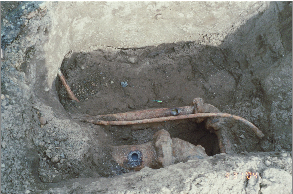
Photograph 12 - Access holes cut in 3-inch-diameter and 6-inch-diameter pipelines in EX-3.
