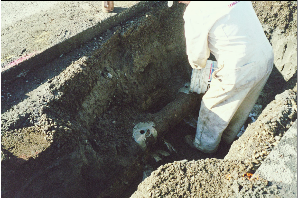
Photograph 9 - Adding grout to 6-inch-diameter pipeline at EX-2.
