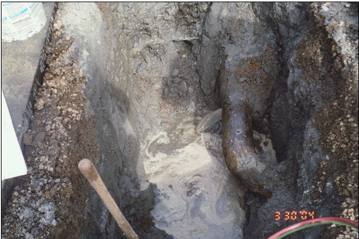
Photograph 8 - Draining accumulated water from 6-inch-diameter pipe exposed in EX-2.
