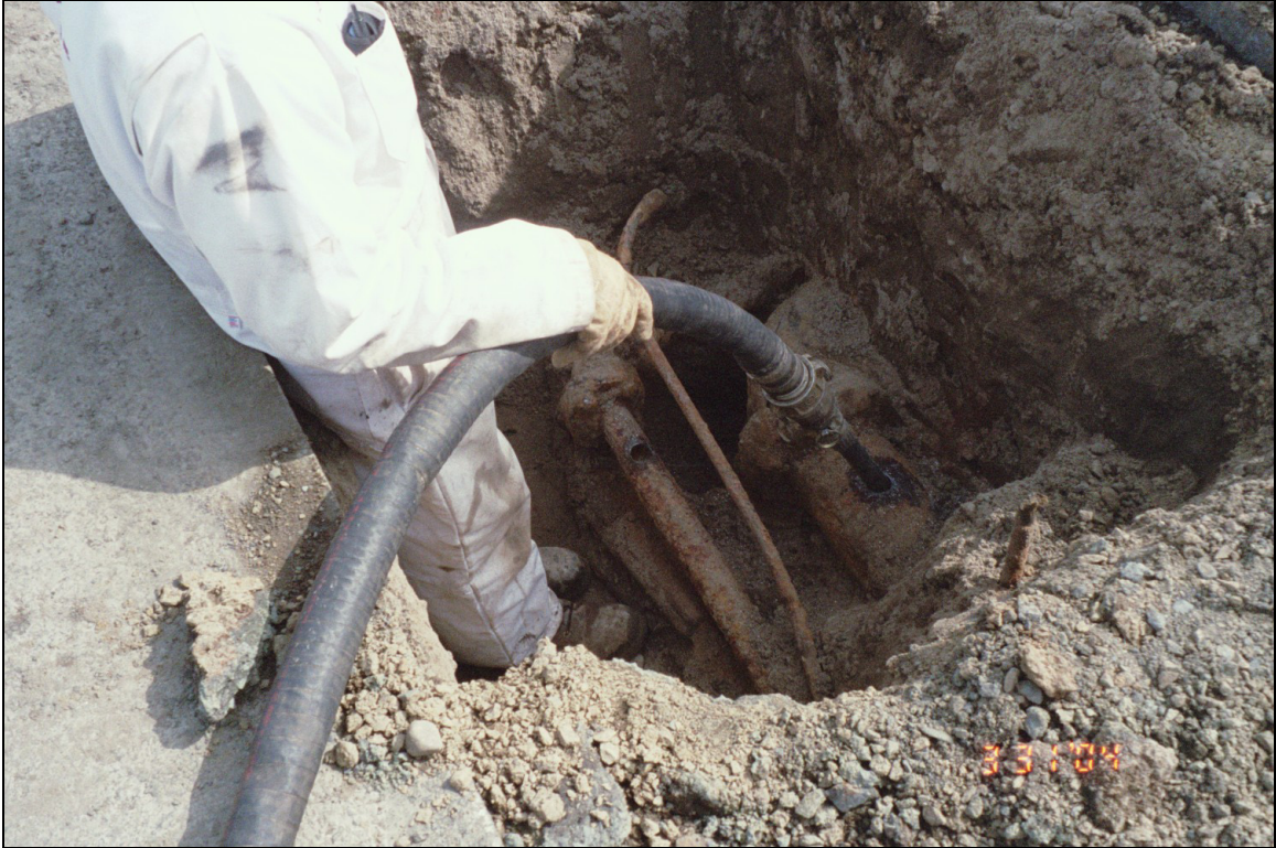
Photograph 13 - Vacuuming emulsified water/product from 6-inch-diameter product line at EX-3.
