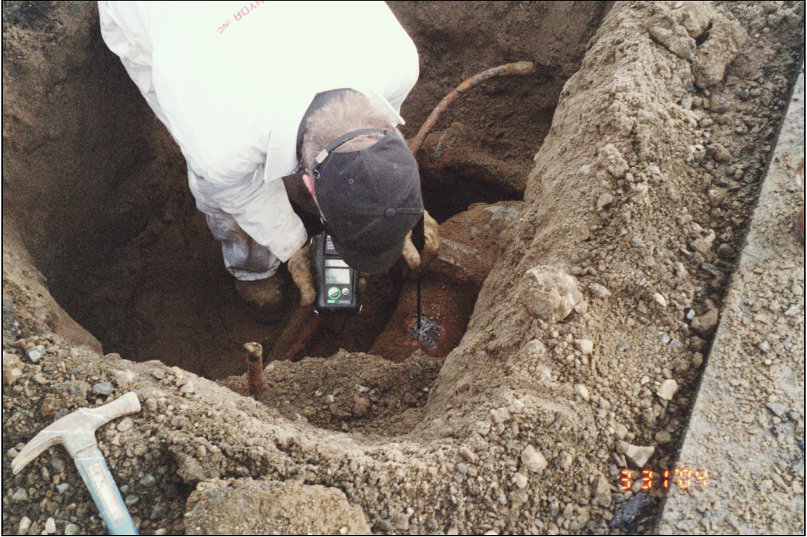
Photograph 11 - Vapor screening 6-inch-diameter pipeline in EX-3.
