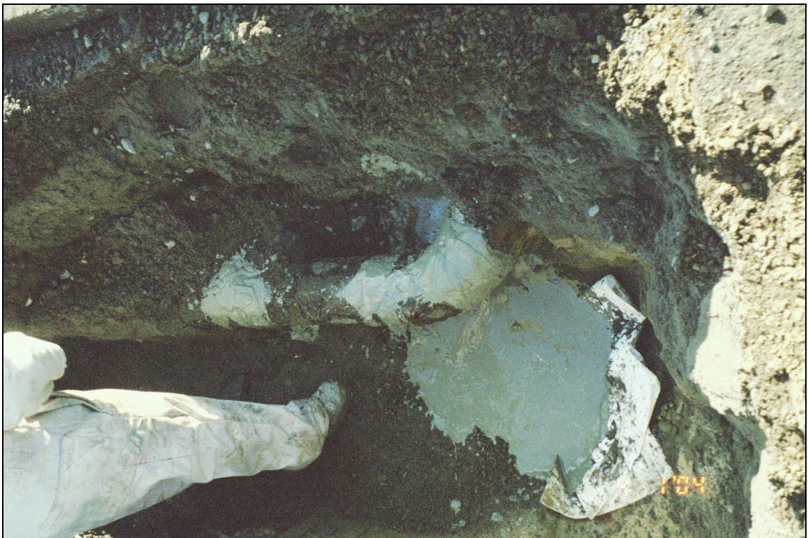
Photograph 10 - Grout seal completed at EX-2.
