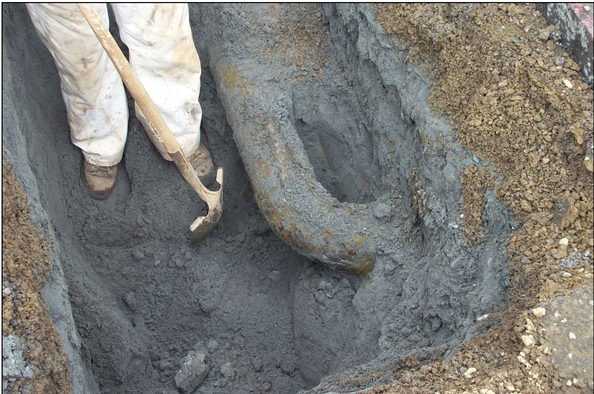
Photograph 4 - EX-2 location showing 90° bend in former Niemi/Mobil bulk plant supply line.
