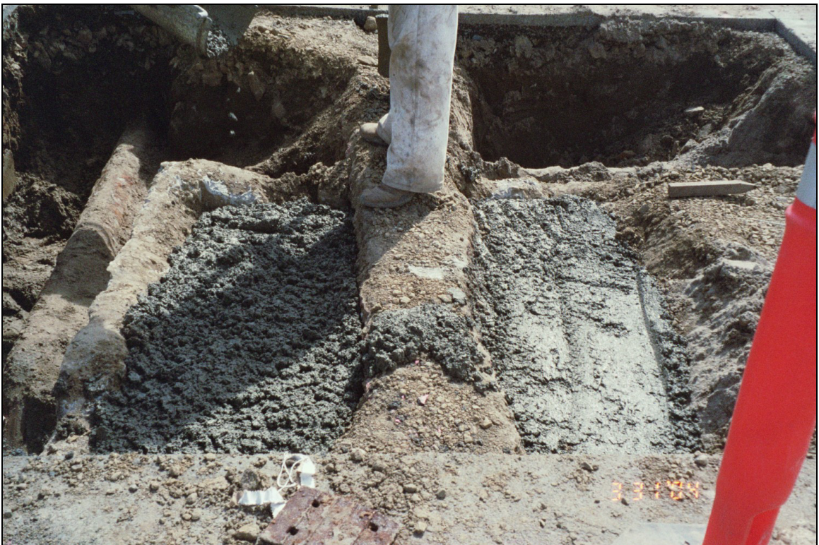
Photograph 16 - Concrete placement in EX-1 vault complete.
