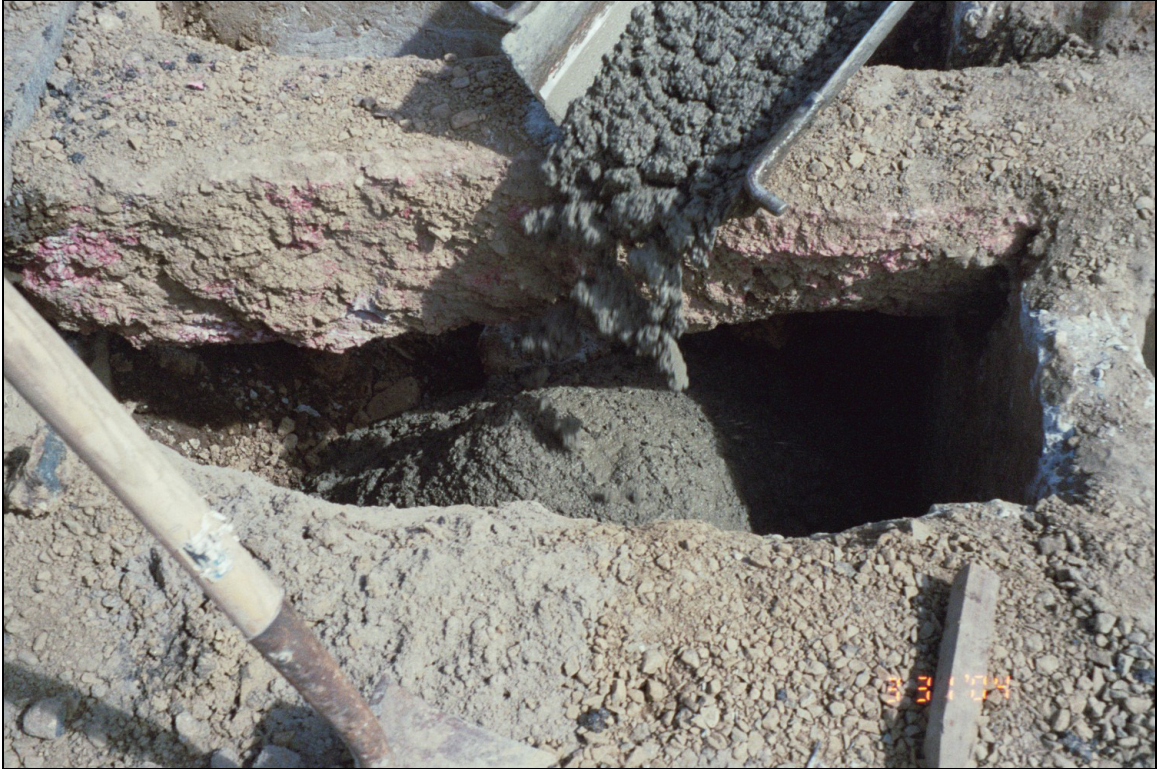
Photograph 15 - Concrete placement in EX-1 vault.
